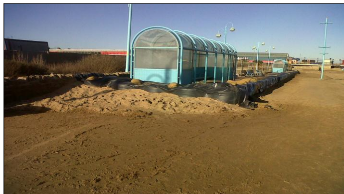
Damage to the Flood wall
