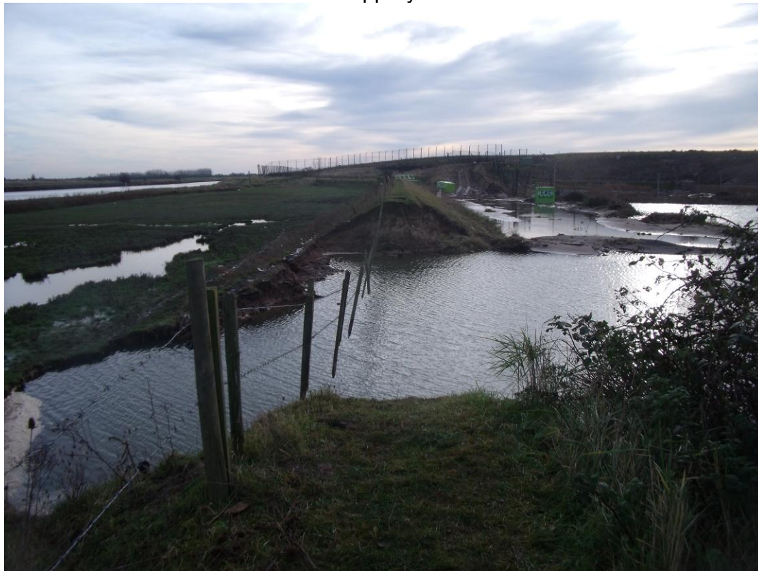
Boston - Breach in sea defence at Slippery Gowt
